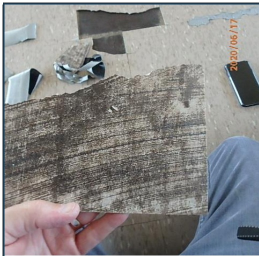
Photo 3: Back of tile showing adhesive pattern
