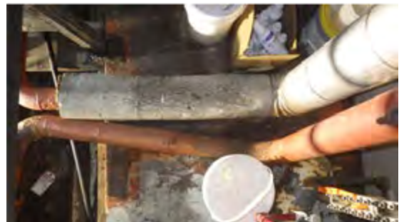
Photo 9: View looking down on pipe segment between vertical coupling and horizontal coupling. Angle of rotation estimated at approximately 7 degrees.
