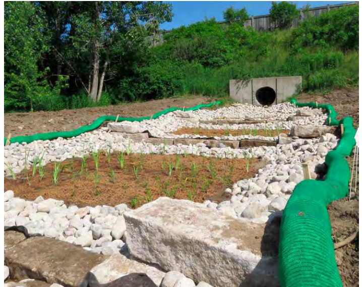
The Pittock biofilter has been planted with 300 native aquatic plants.
