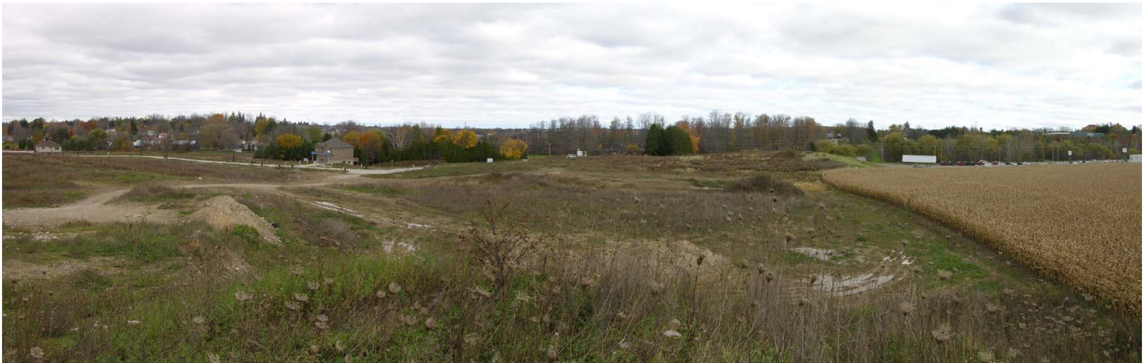
View of eastern section of subject site - looking to Harris Street (Oxford Road 119)
