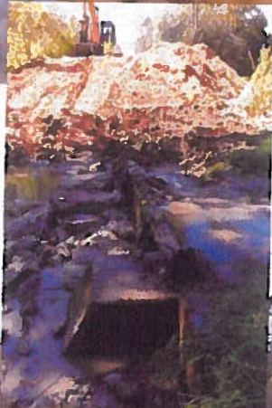
Above: The last pieces of the dam to be removed after two years of gradually demolishing the structure. Right: The remaining barrier is removed in September 2014. Below: Tree planting next to the stream, free-flowing after 46 years.
