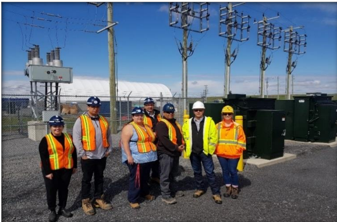
Photo 6: Tour participants in front of facility where electricity made from landfill gas enters the grid.
