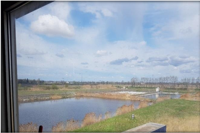
Photo 4: Storage ponds for leachate and storm water post treatment process, prior to discharge.
