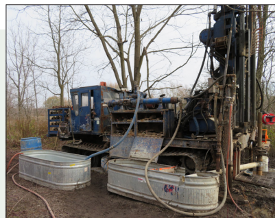
Drilling for groundwater monitor well installation.
