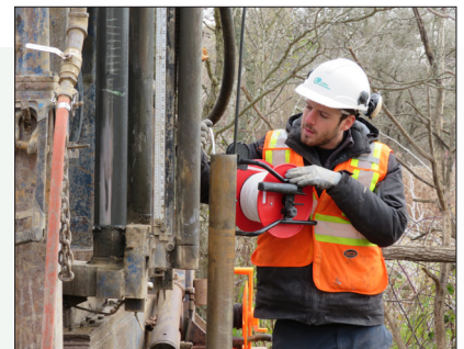
Checking depth of groundwater monitor well for installation.
