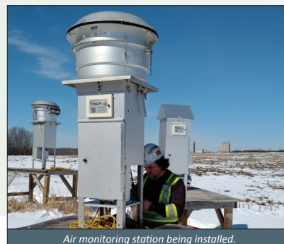
Air monitoring station being installed.
