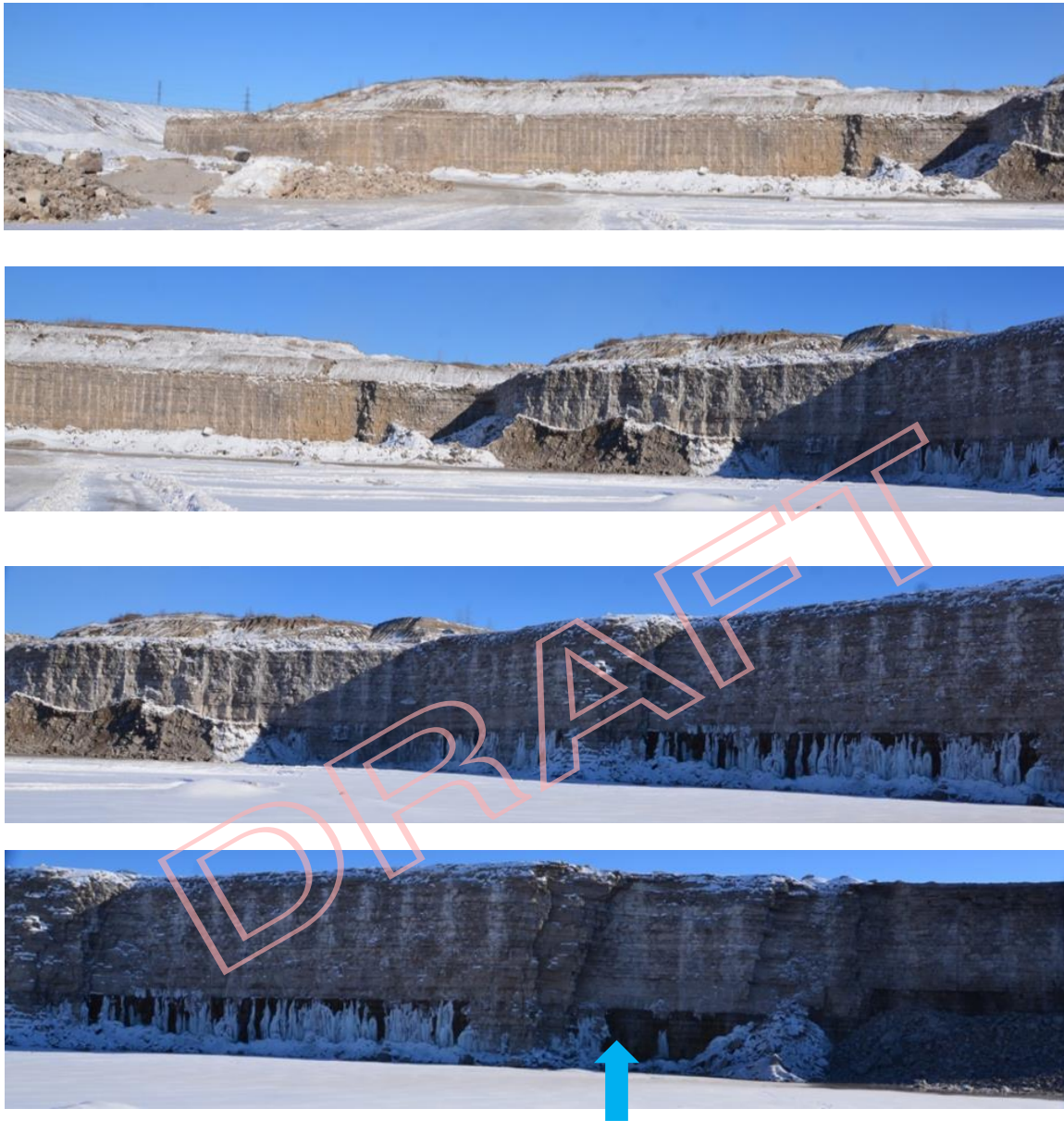
Figure 6. Overlapping panoramic views of the east and south faces of the active quarry, showing negligible groundwater flow from the east face (top photo) and distributed flow along the length of the south face (bottom photos). The blue arrow shows the location of the largest inflow to the south face. A close-up of the inflow is shown in Figure 9.
