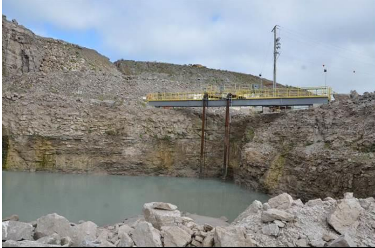
Figure 5. Looking west to the sump in the active quarry. The water surface is ~230 m above sea level. This is the lowest point in the quarry and so there is groundwater flow towards the sump from all directions. The north side of the sump pool has the largest preferential flows into the pool. Most of the water emerges from a single bedding plane, where the largest aperture is probably several millimetres. Nearby blasting activities may have resulted in fracture enlargement here.
