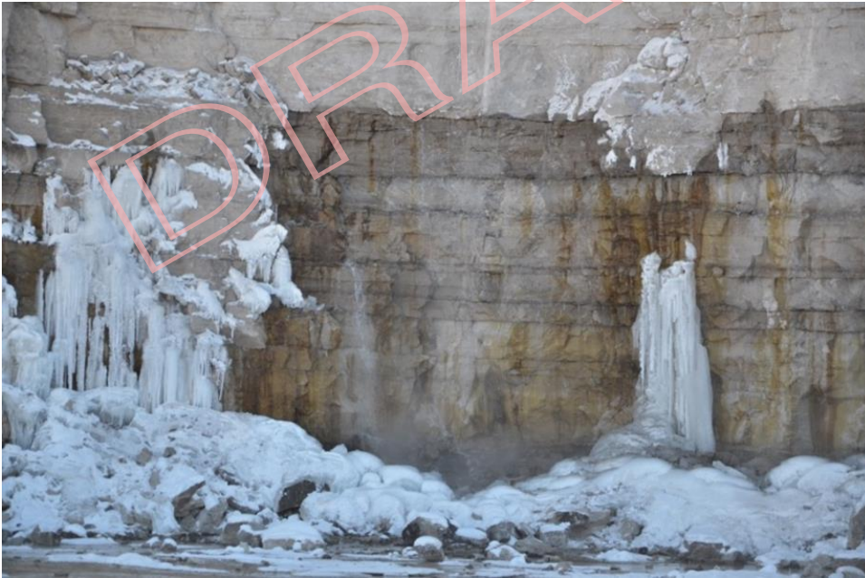
Figure 9. Views of the two largest discharges from the quarry face observed on the visit of February 1, 2019. (Top) A point discharge into the quarry sump. The same location is also shown in summer in Figure 5. (Bottom) A point discharge from the south face. The location is shown by the blue arrow in Figure 6.
